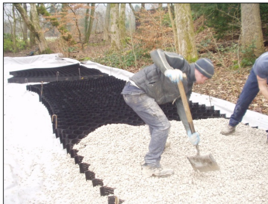
Photo 3- expanding and filling the Cellweb system
