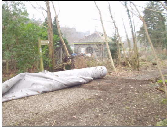
Photo 2- laying of Fibretex material onto existing subgrade
